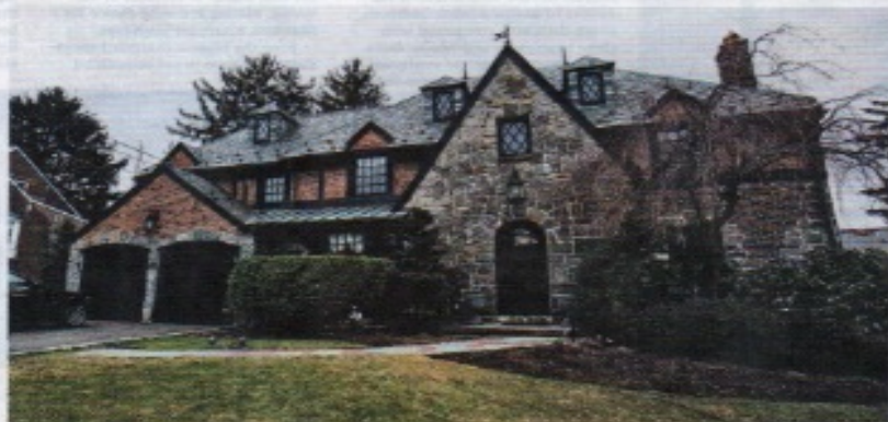
ORIGINAL CONDITION To keep the facade of the house the same after the renovation, owner Anthony Faglione used brick and stone reclaimed from other homes that were demolished but came from the same era.
